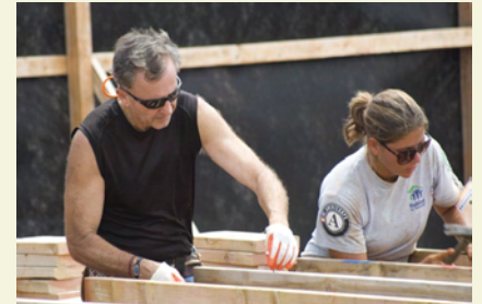
Steve Latham and Hannah Livingston installing blocking.
