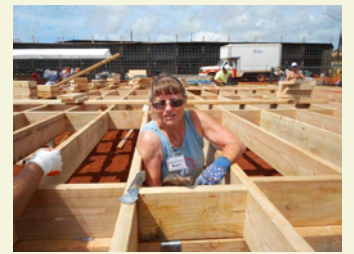
Kaye Leonard installing hurricane straps.
