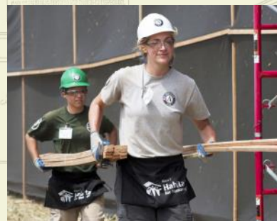
Team leader Alicia D'Allesandro (left) and Briana Kasman (right) work to finish dust fence construction at the 'Eleele 'Iluna Subdivision. (June 2013)
